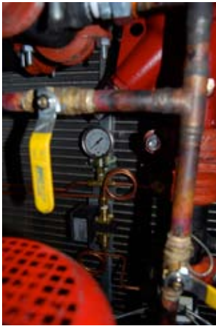
Factory Installed Pressure Gauges and Shutoff Valves
